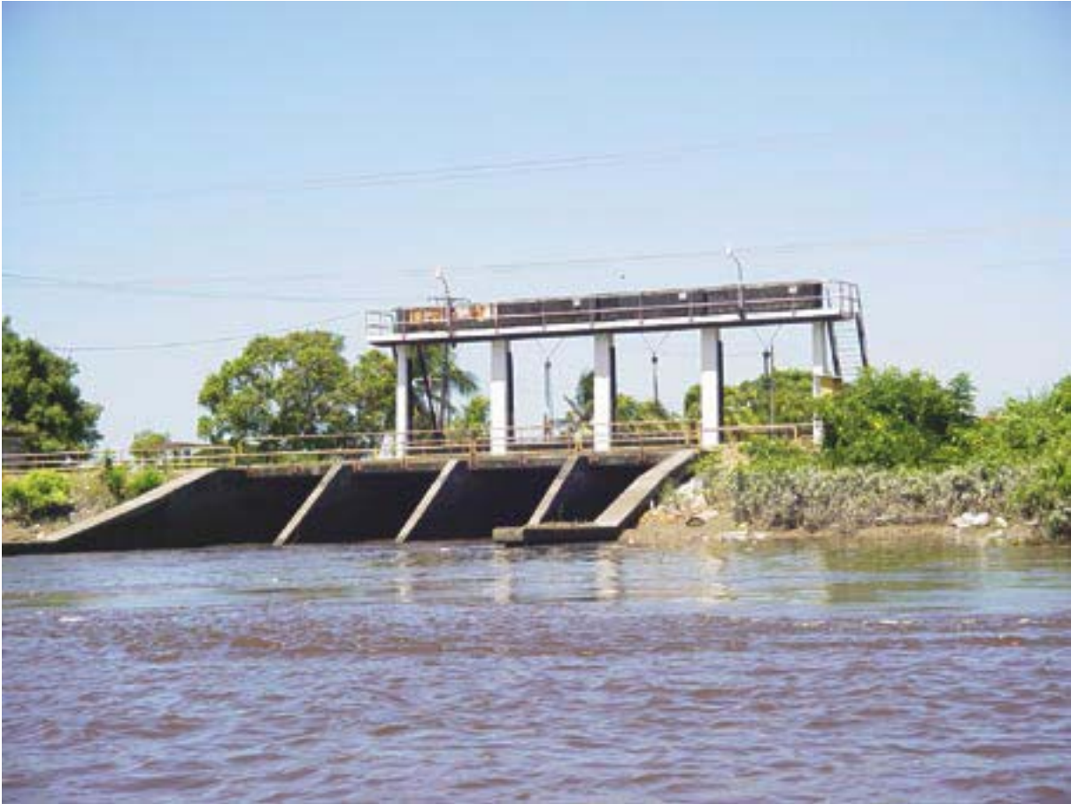
Picture 4-5: Drainage outlet in the Nickerie river (2004)
